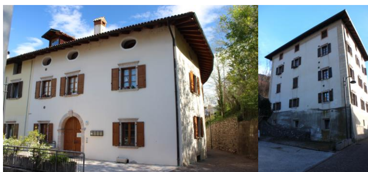
Figure 12: On the left ex casa Bortoli, on the right the isolated building.
